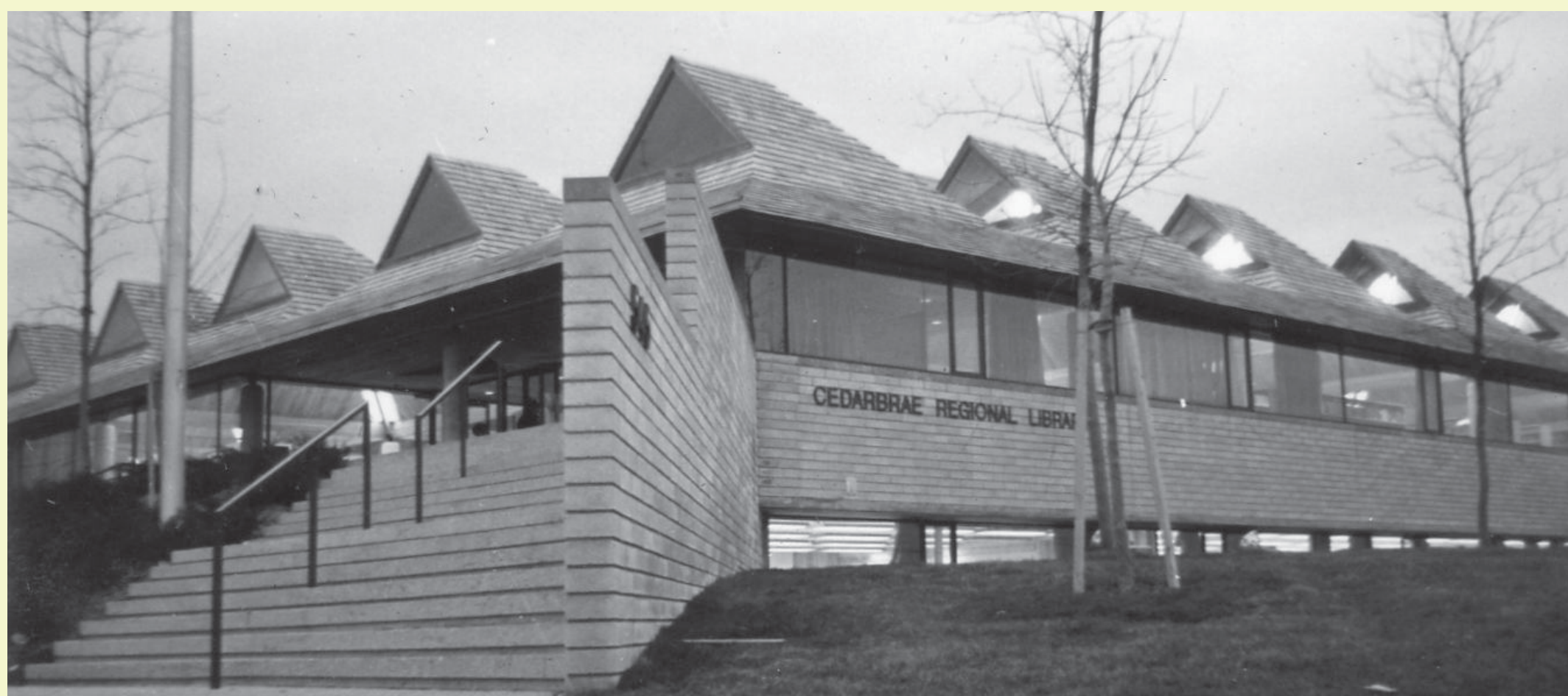
Cedarbrae Regional Library, autumn 1966. Architect Irving Grossman placed the library "in as dramatic a way as possible," so it would be a focal point of the community. The main entrance was on the upper level, accessed by a concrete ramp from the east parking lot and a steep angled concrete stair from the northwest.
